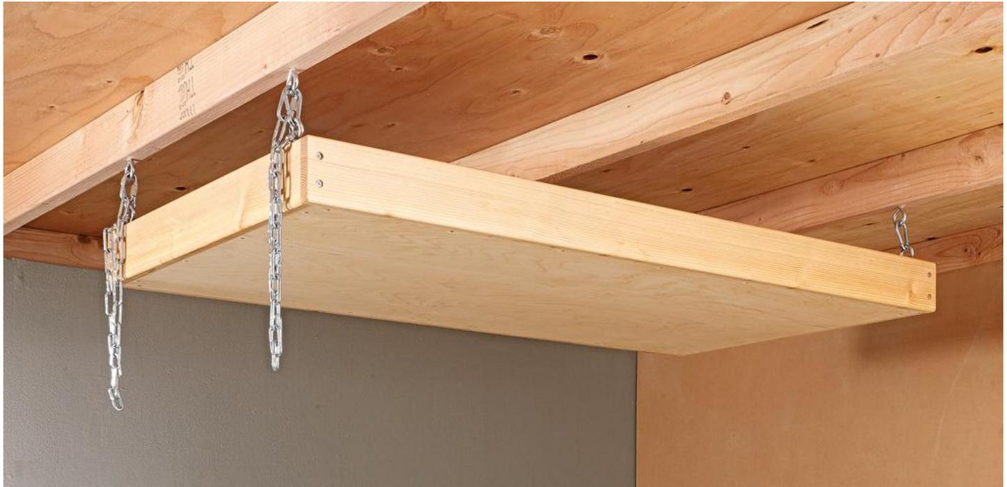
Connecting the snap links with the rafter-mounted eye bolts holds the tray closed. Both front corners of the tray, however, also have a short length of chain that's connected between the eye bolts with quick links. To access the tray, release the snap links and gently lower the tray until it's supported by the chains.
